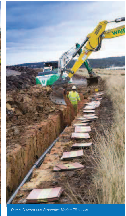
Excavate Trench. Subsoil Store separate to topsoil store and lay ducts
